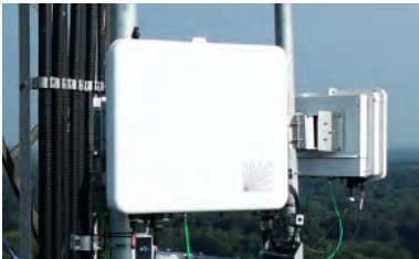
Tarana G1 Base Nodes (BNs) on Vertical Asset
